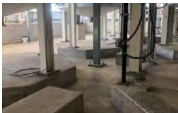
Typical medium-corrosive environment — exterior anchorage.
