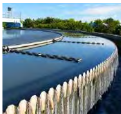
Typical severe-corrosive environment — wastewater treatment plants.
