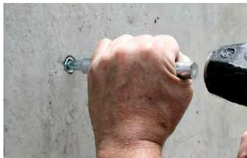
Anchor being set with hand setting tool.
