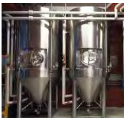
Typical high-corrosive environment — food-processing plants.
