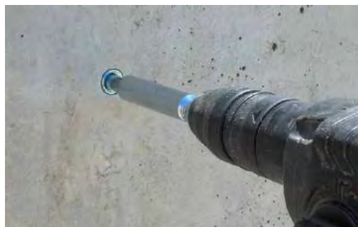
Anchor being set with SDS setting tool.
