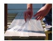
If the board is damaged on both sides, please set the board aside for replacement. The installation of a damaged board is not covered under the Aeratis Warranty.
